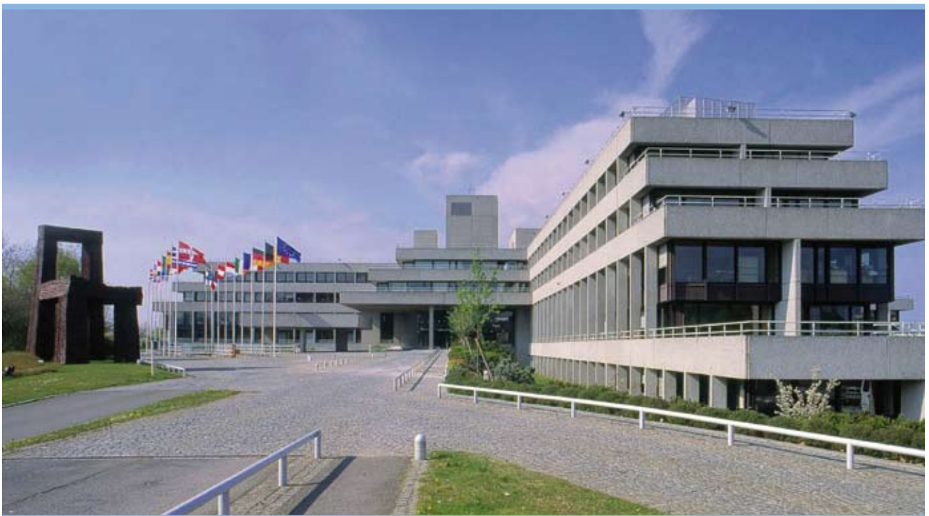
The EIB's first permanent building was designed by Sir Denys Lasdun. The chair sculpture by Magdalena Jetelová was installed in 1999.
