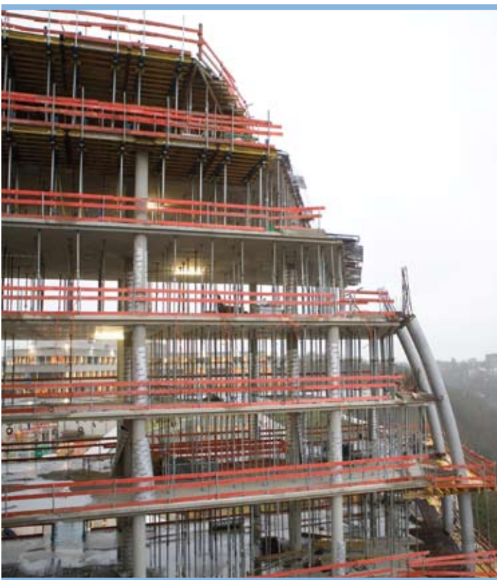
Another work in progress shot taken in December 2006.
