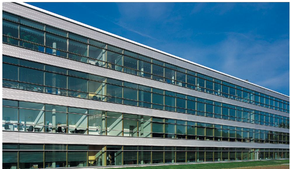
Holz-Metall-Elementfassade HMEF 2020 timber unitised curtain wall HMEF 2020
